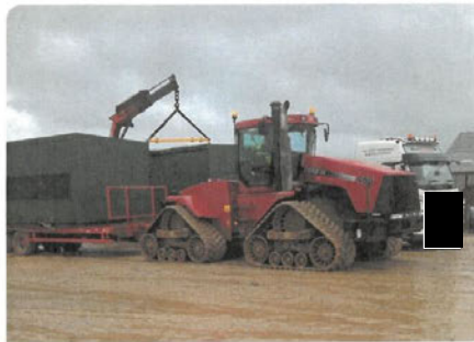
Case Steiger Quadtrac used to deliver inverters and other heavy equipment to site under soft ground conditions (photo courtesy of British Solar Renewables)
