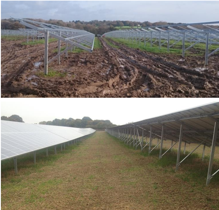
Inserts 26 and 27: Inter-row Ground Restoration
