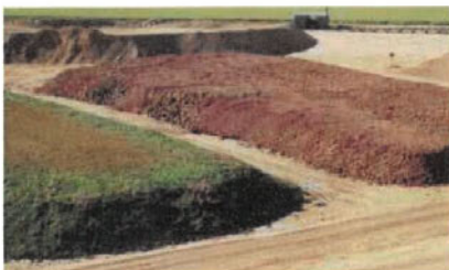
Clearly defined stockpiling of different soil materials
